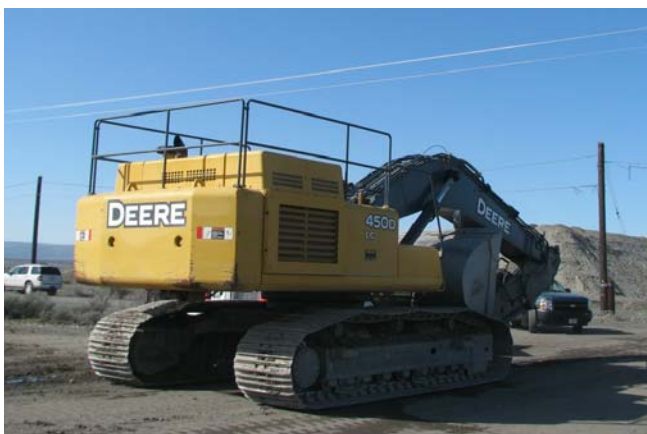
Figure 1 - Excavator that touched energized power line
