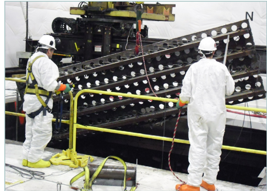
Figure 2-3. Workers at Brookhaven National Laboratory (BNL) load neutron shield pieces from the Brookhaven Graphite Research Reactor (BGRR) into a shielded container for shipment to a disposal facility. BNL submitted lessons learned in 2011 that involved BGRR.
