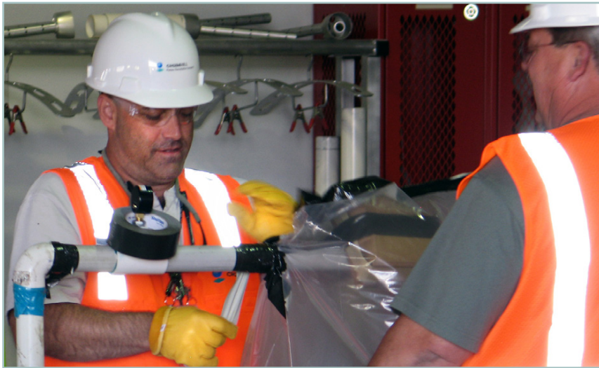
Figure 1-1. New D&D hires practicing containment wrapping
