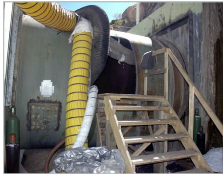
Figure 2-3. Access door cut into penstock for recoating work
