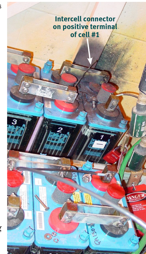
Figure 2-3. Connection of cells 1 and 120 and aftermath of arc flash
