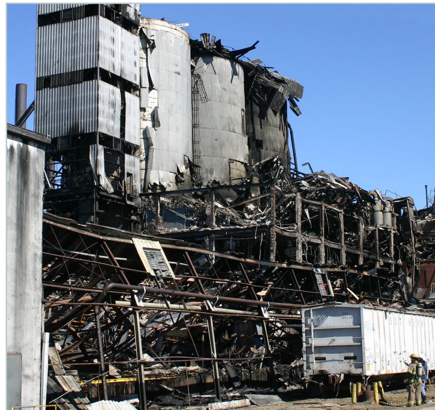
Figure 2-1. Elevator building, silos, and packing facility following explosion and fire
