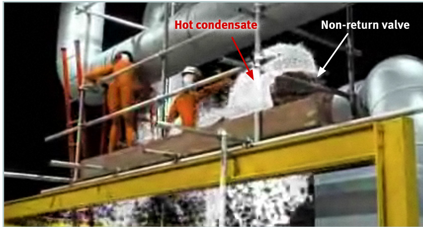
Figure 1-5. Workers engulfed in hot condensate on scaffold (animation) (Source: Rye House video)
