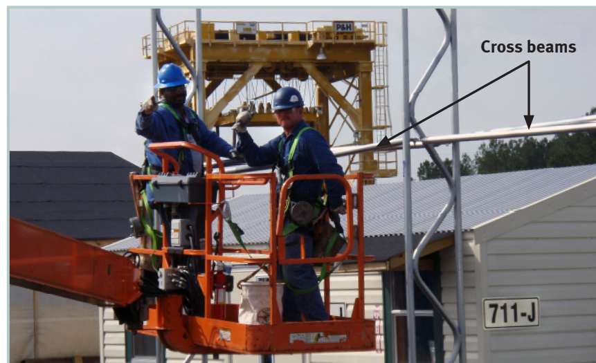
Figure 2-1. Lift basket and cross beam
