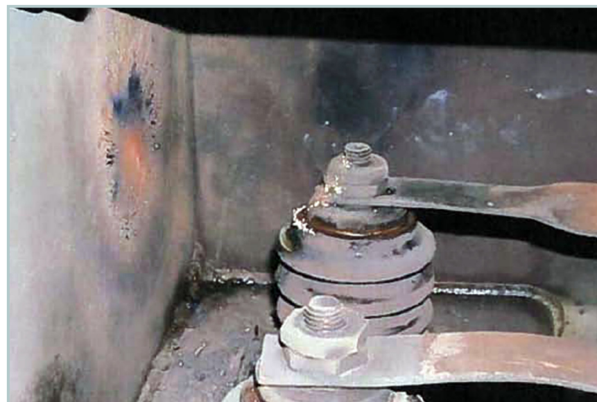
Figure 1-2. Damage to cabinet from arc flash
