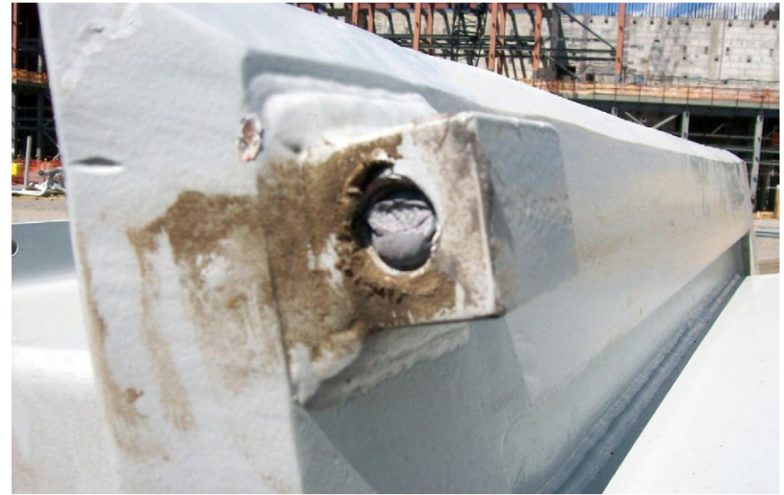
Figure 1-6. Installed eye nut not shouldered to the flange
