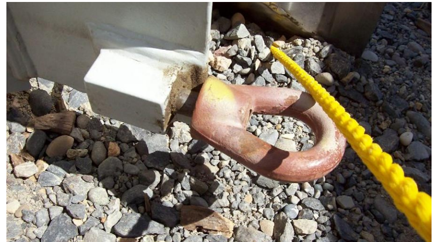
Figure 1-7. One of the four lifting flanges on the liner with a broken stud
