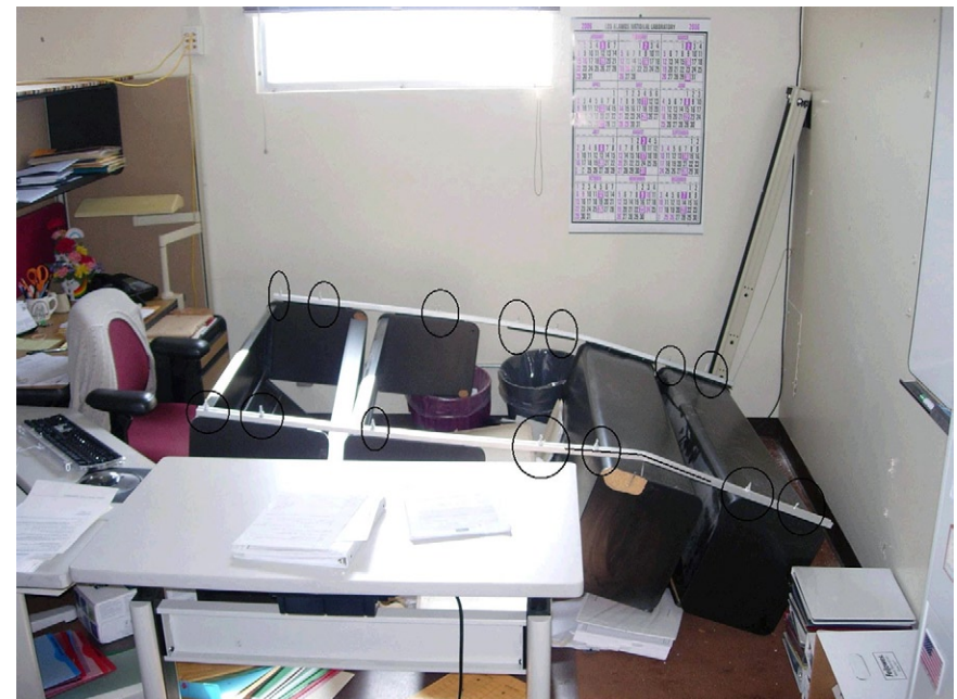
Figure 1-3. Fallen office shelving (anchors are circled)
