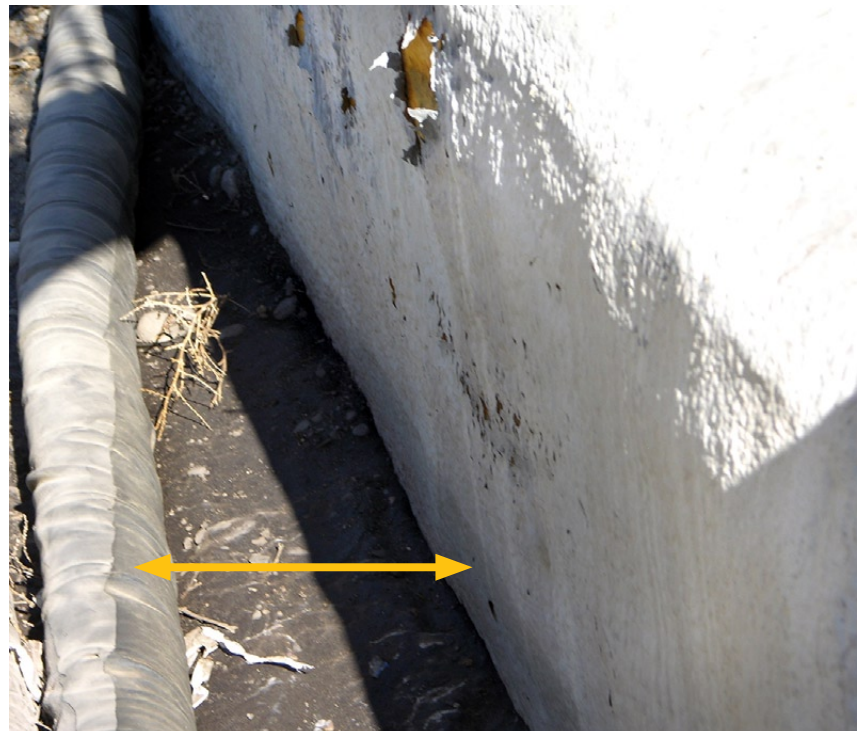
Figure 2-1. Double-sided arrow shows “bathtub ring” along the top of the hose and on the pump pit wall
