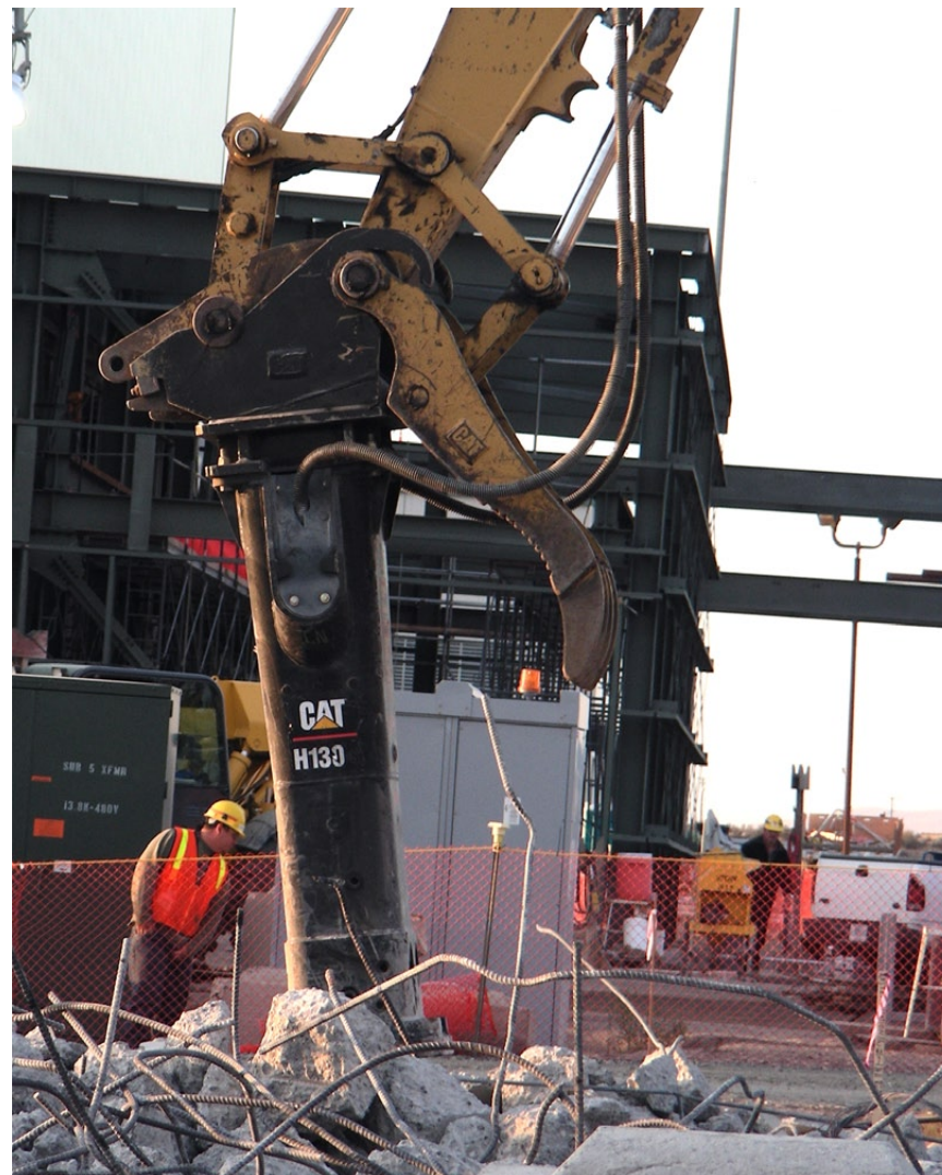
Figure 1-1. Hydraulic hammer attachment at location of rebar and concrete debris
