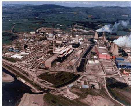
Figure 3-1. Thermal Oxide Reprocessing Plant
