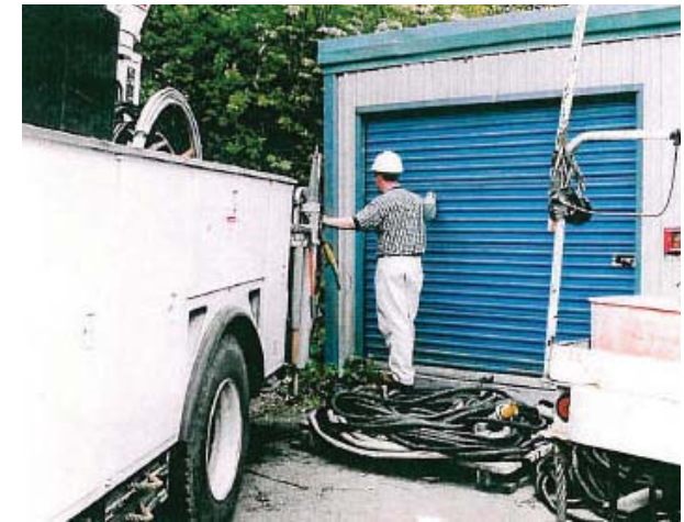
Figure 2-2. Incident reenactment (touching the energized truck and the grounded metal building)
