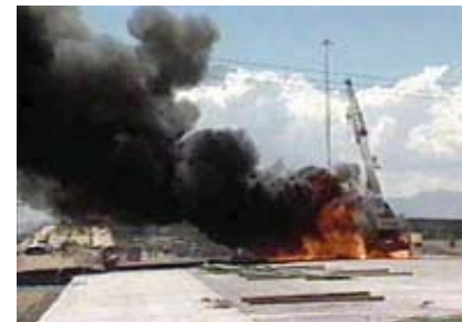
Figure 3-1. Crane cable contacts 7,200-volt power line (Source: OSHA website)
