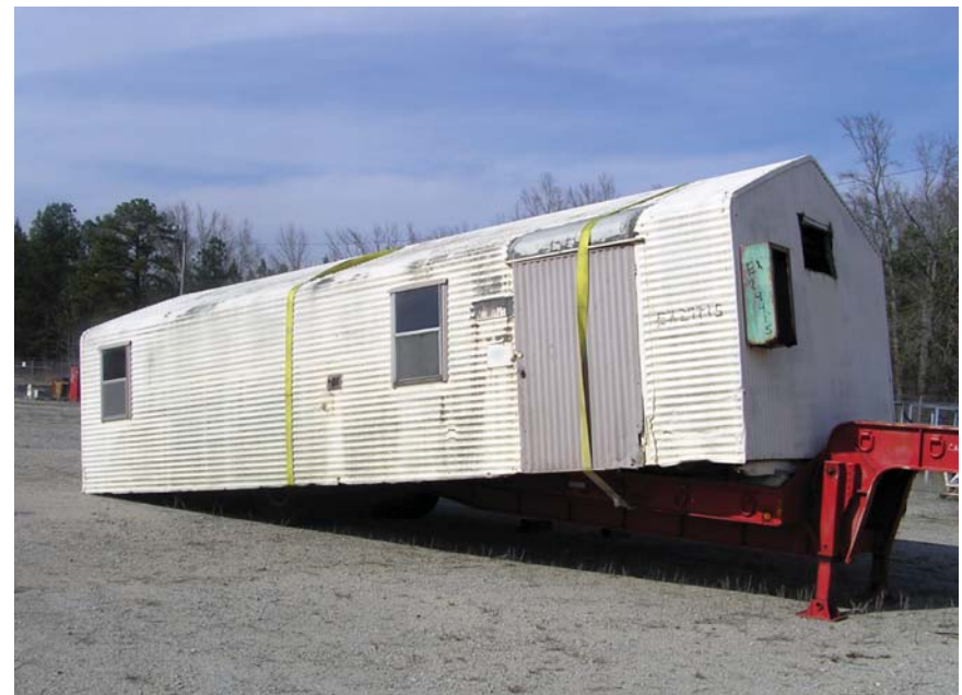
Figure 1-1. Portable building that collapsed
