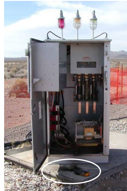
Figure 1-1. Pump motor controller and damaged meter on concrete pad (circled)
