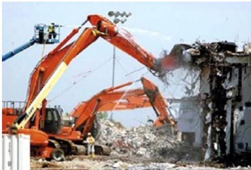
**Figure 3-2. Dust control during demolition**
