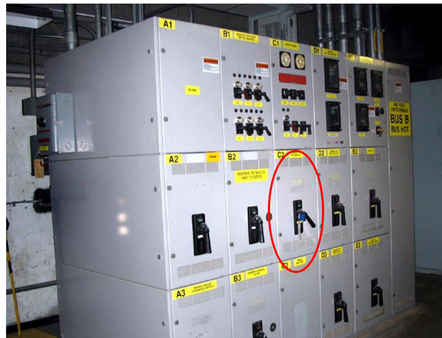
Figure 2-1. Motor Control Center with the 480-volt circuit breaker (circled in red)
