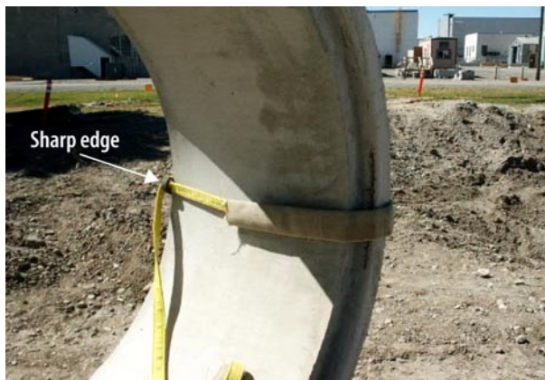
Figure 1-2. Lifting sling configuration
