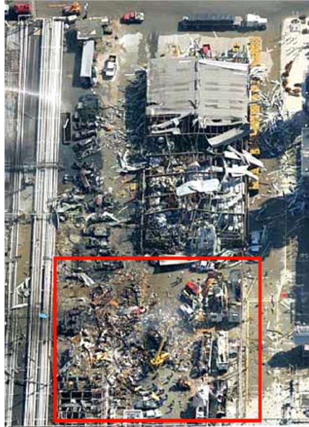
Figure 3-2. Destroyed temporary trailers (red box)
