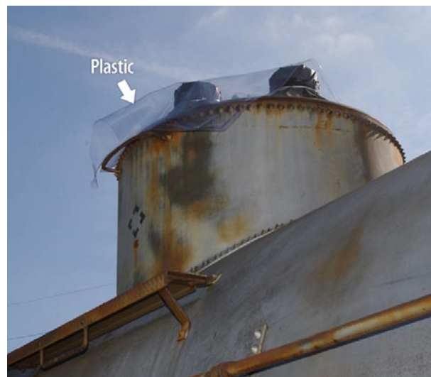
Figure 4-1. Plastic on rail tank car hatch
