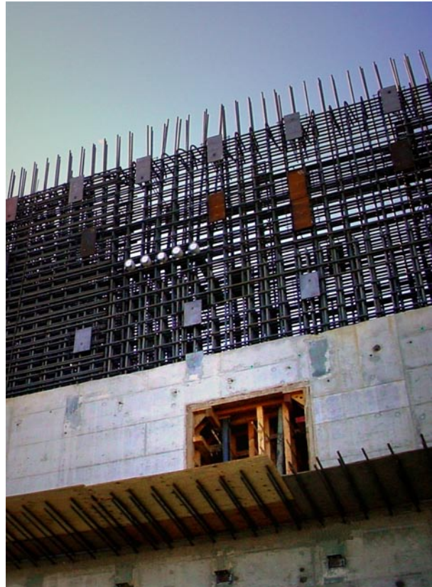
Figure 4-1. Rebar wall
