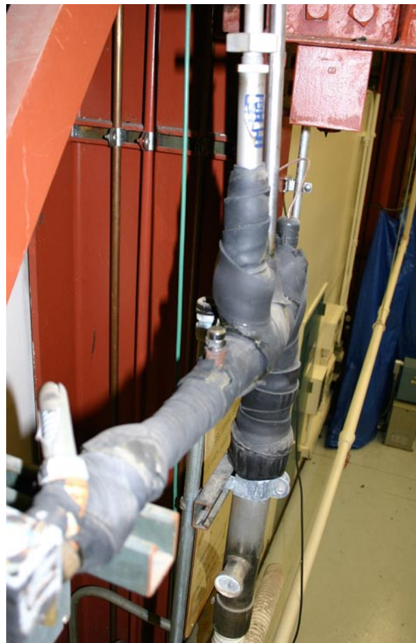
Figure 3-1. Pressure relief valve
