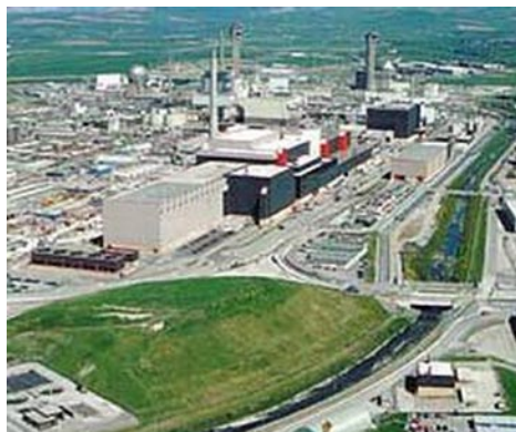
Figure 4-1. Thermal Oxide Reprocessing Plant
