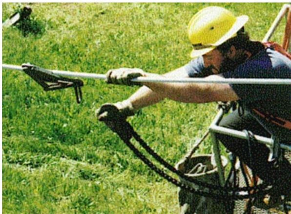
*Figure 3-4. Reenactment of lineman removing gripper from conductor*
