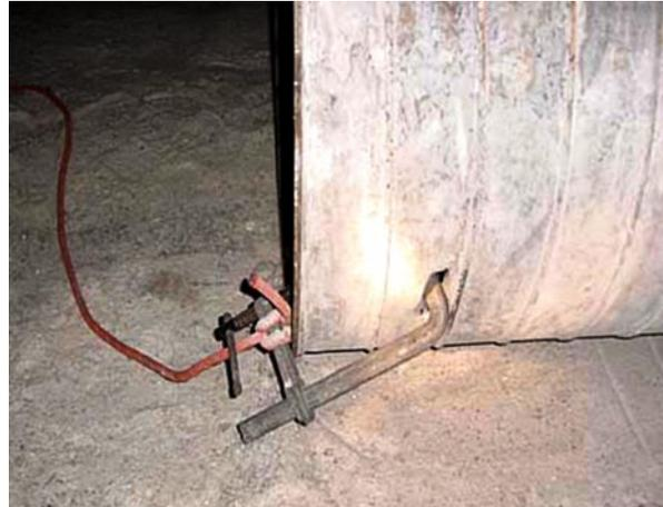
*Figure 2-2. C-clamp attached to vent line*
