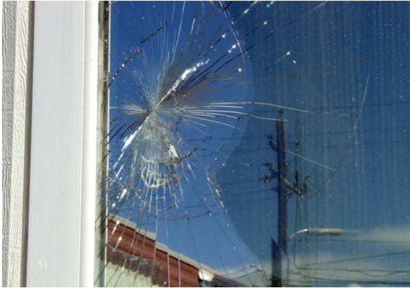
Figure 3-2. Shattered window on trailer
