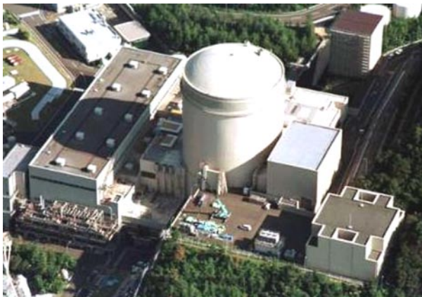
Figure 1-1. Turbine building to the left of the reactor building (center)
