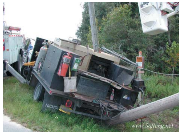
Figure 1-3. Truck and top section of utility pole
