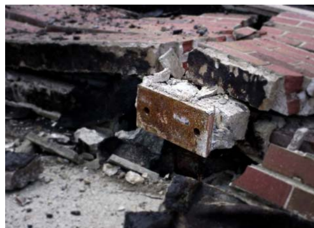
Figure 1-3. Unsecured base plate
