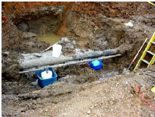
Figure 1-1. Typical LLWP pipeline
