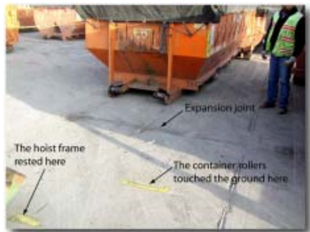
Figure 2-2. The container and concrete on which it rested
