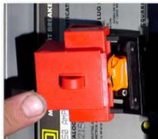
Figure 5-3. Reenactment showing lockout device installed with electrical tape (orange) applied to circuit breaker handle
