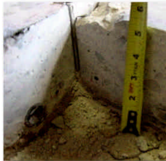
Figure 1-2. Cut conduit (left) crossing into corner of the cut area
