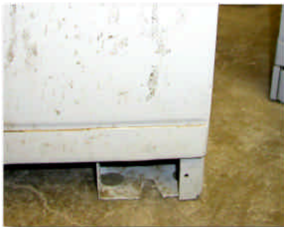
Figure 1-3. Mounting hole in cabinet base
