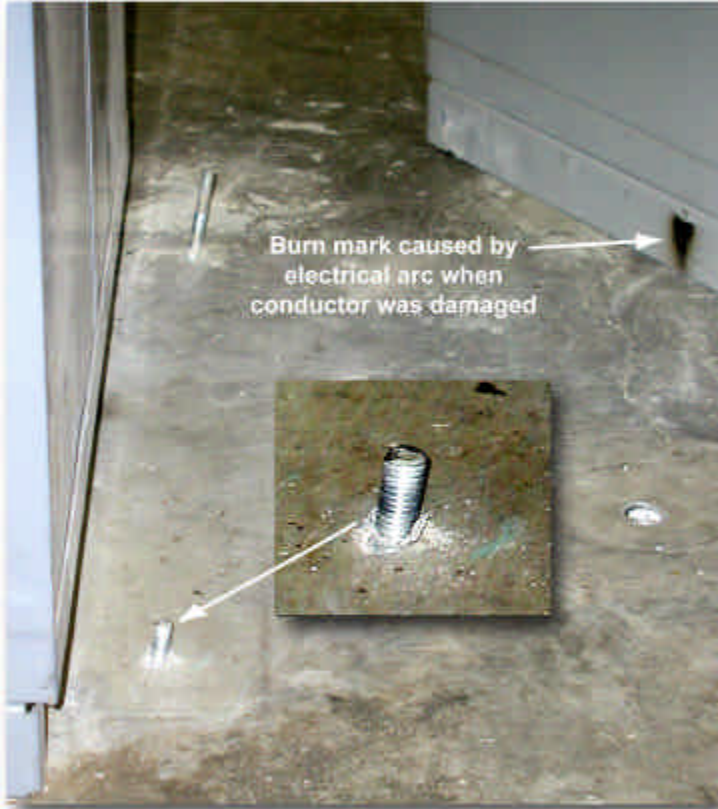
Figure 1-2. Enlarged view of the floor anchor and cabinet
