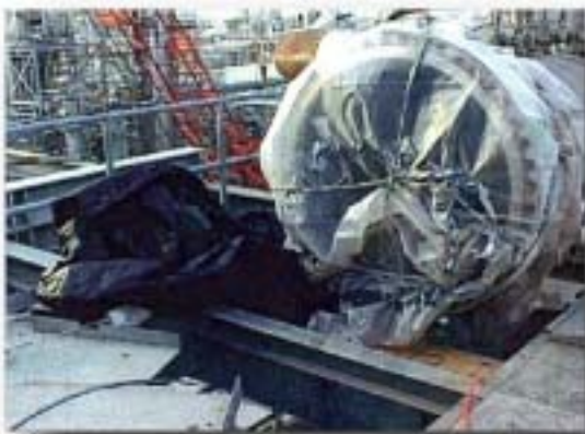
Figure 4-1. Pipe where workers were overcome by nitrogen-enriched atmosphere
