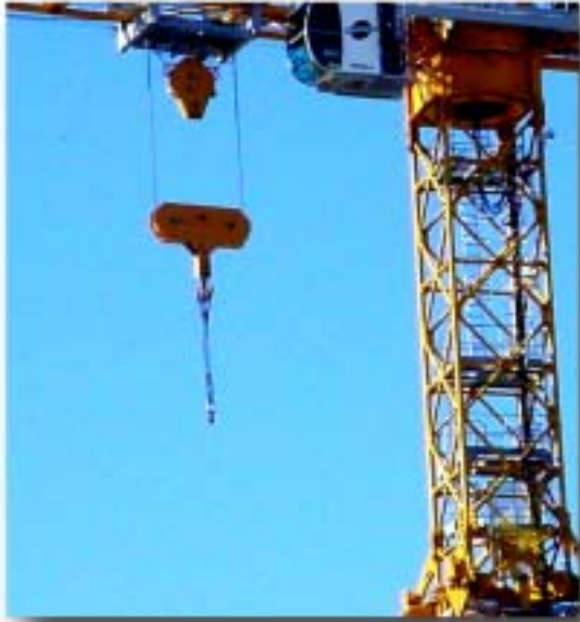
Figure 3-2. The tower crane with its rigging
