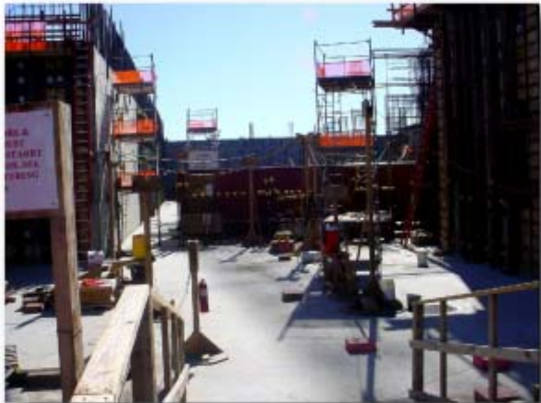
Figure 3-1. The congested construction site
