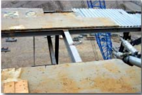
Figure 4-3. Roof opening near the skiff box
