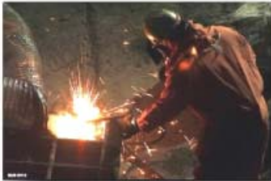
Figure 4-1. Typical torch cutting operation
