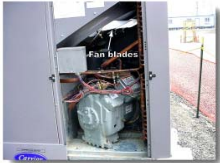
Figure 4-2. Compressor with fan blades above
