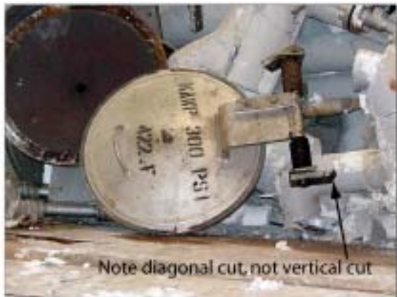
Figure 5-1. The lid and hinge bracket
