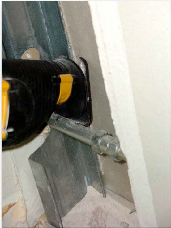
Figure 2-1. The boot of the saw resting against the conduit
