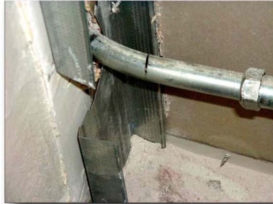
Figure 2-2. The cut conduit
