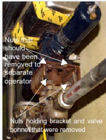
Figure 1-1. The air-operated valve configuration
