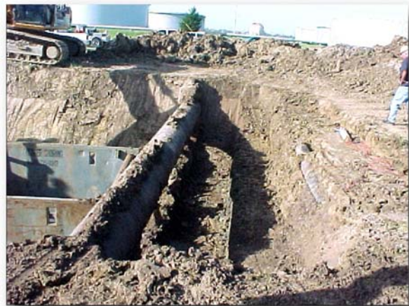
Figure 1-2. The excavation after the slope was corrected
