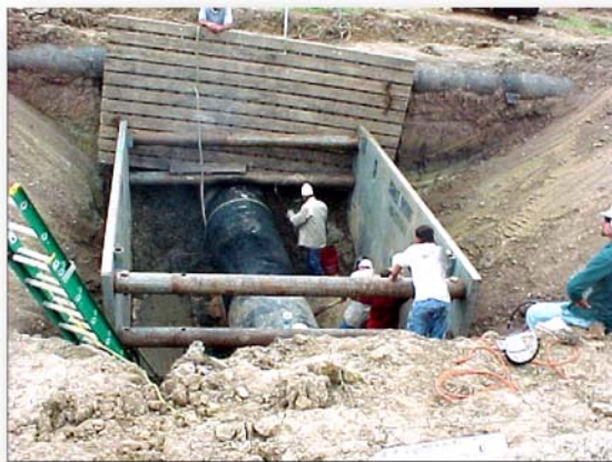
Figure 1-1. The original placement of the trench box in the excavation
