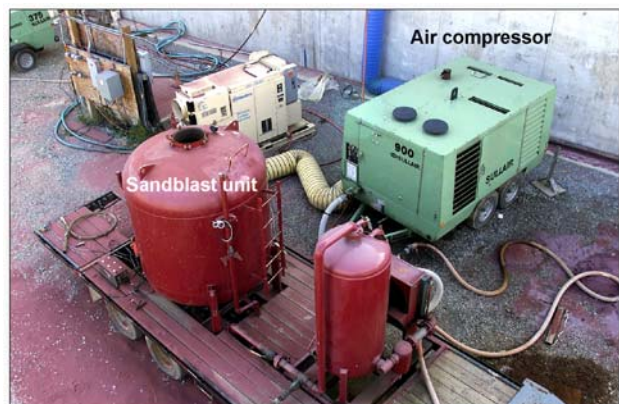
Figure 3-2. Sandblast unit next to air compressor
