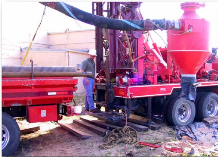
Figure 1-1. Truck-mounted drill rig
