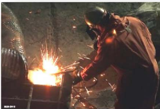
Figure 2-1. Torch cutting at Fernald
