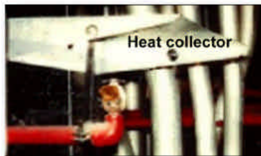
Figure 5-1. An upright sprinkler with a heat collector
