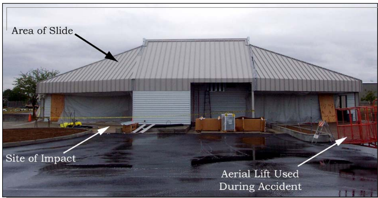
Figure 2-1. Building 960 construction site
