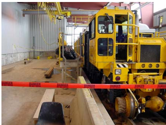
Figure 1. A view of the platform and trackmobile
