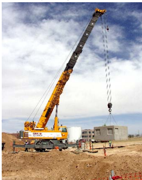
Figure 1. Crane lifting the manhole structure
