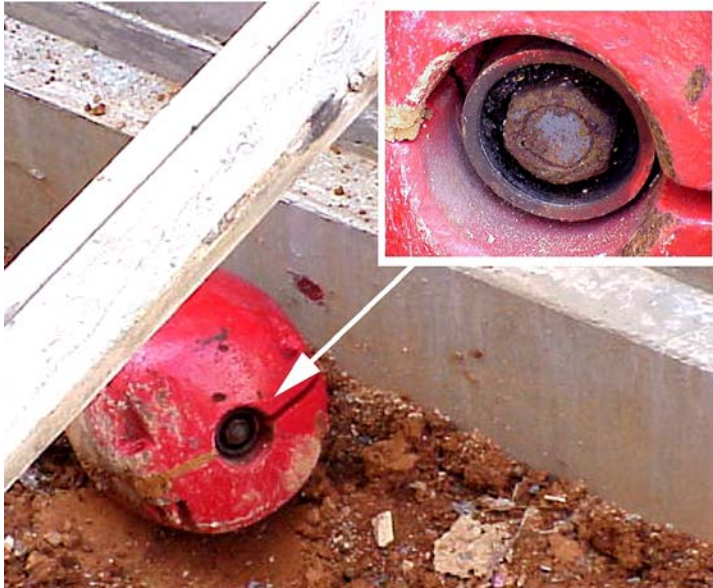
Figure 1. Fallen headache ball and connection threads (insert)
