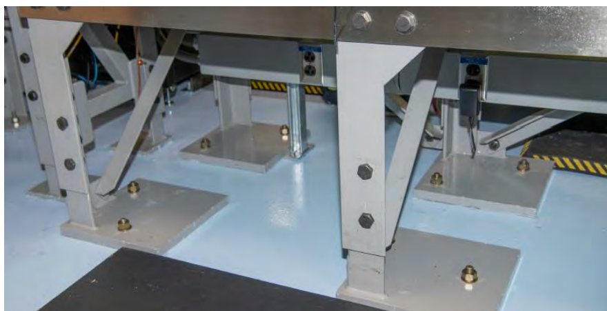
Figure 9: Seismically qualified glovebox stand used for operations with molten plutonium.
