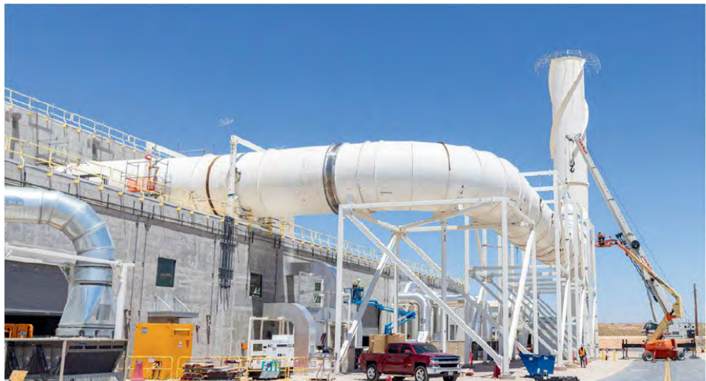
Figure 53. Safety Significant Confinement Ventilation System filtration building and exhaust stack.
