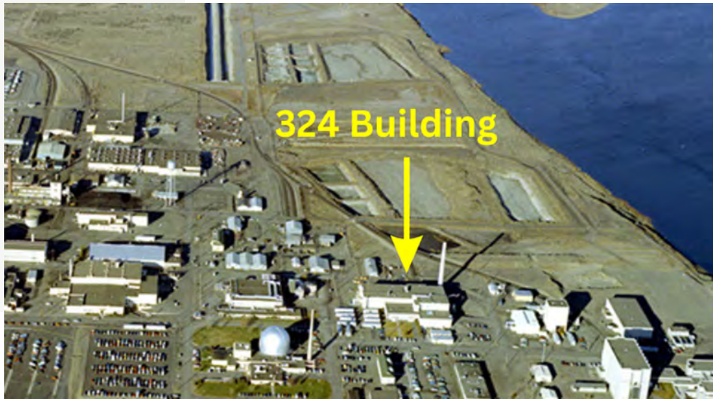
Figure 22. Building 324 in relation to Columbia River.
