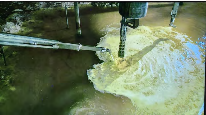
Figure 19. Waste retrieval operations at Hanford Tank Farms.
