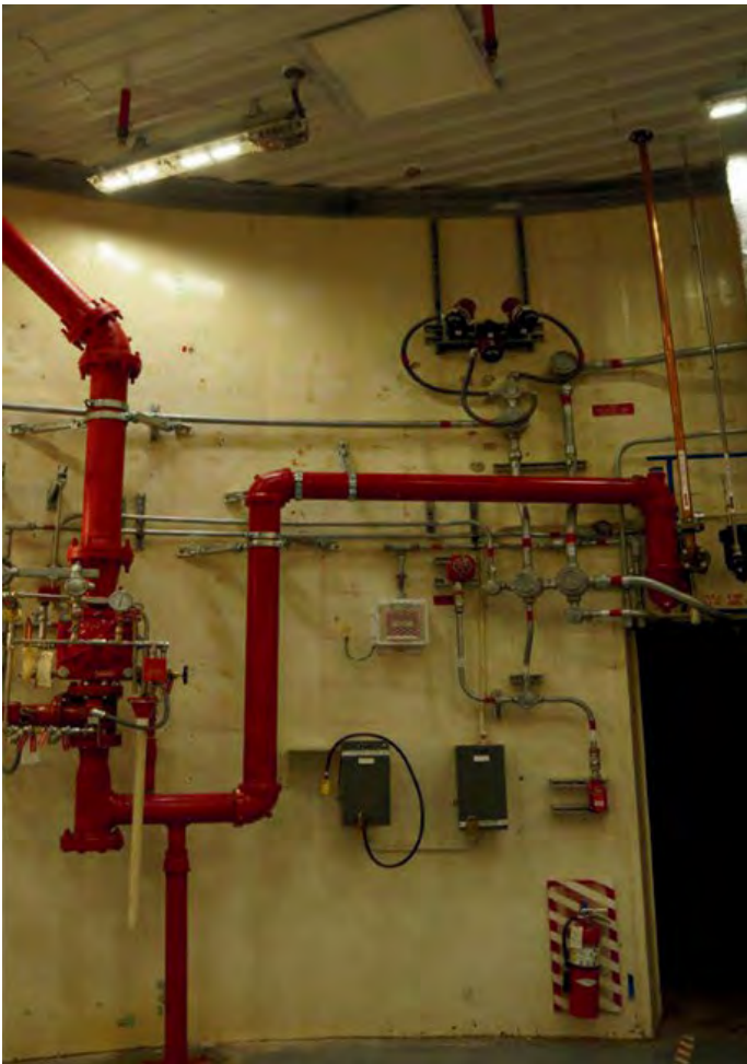
Figure 2. 12-44 cell fire suppression deluge riser where cast iron fittings were installed.
