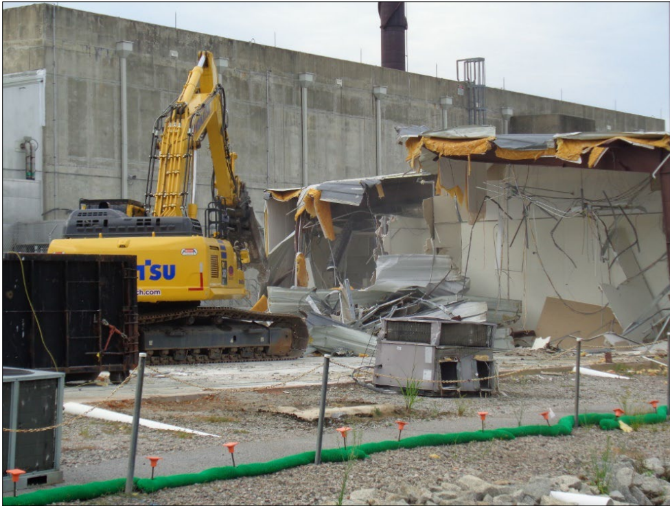
Figure 5. Demolition Activities Supporting Site Preparation for the Tritium Finishing Facility
