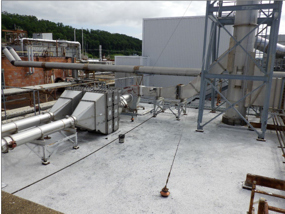
Figure 24. Y-12 Building 9215 Roof Remediation
