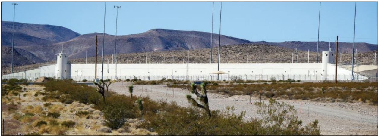
Figure 8. Device Assembly Facility at the Nevada National Security Site
