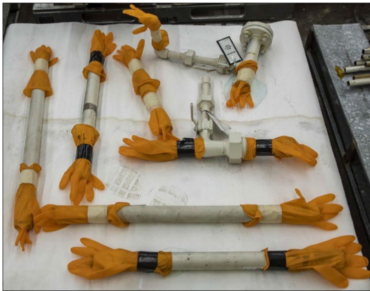
Figure 6. Machine Coolant Piping Capped with Rubber Gloves
