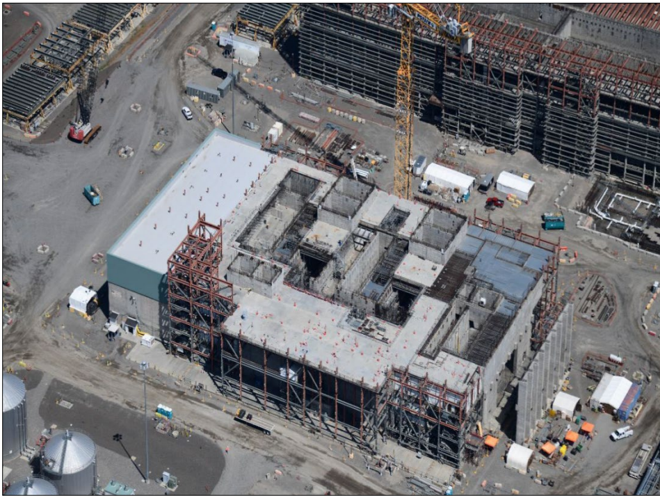
Figure 18. High-Level Waste Facility Construction
