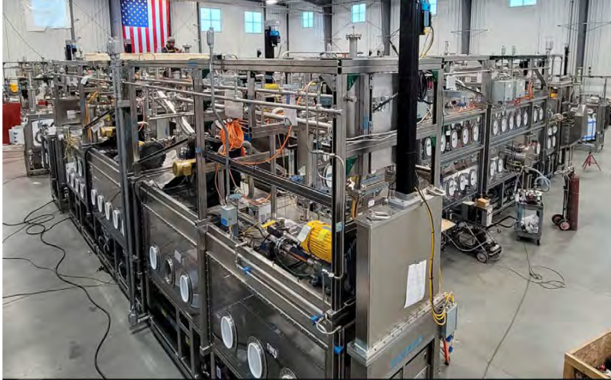
Figure 21. Glovebox line manufactured at a vendor facility.
