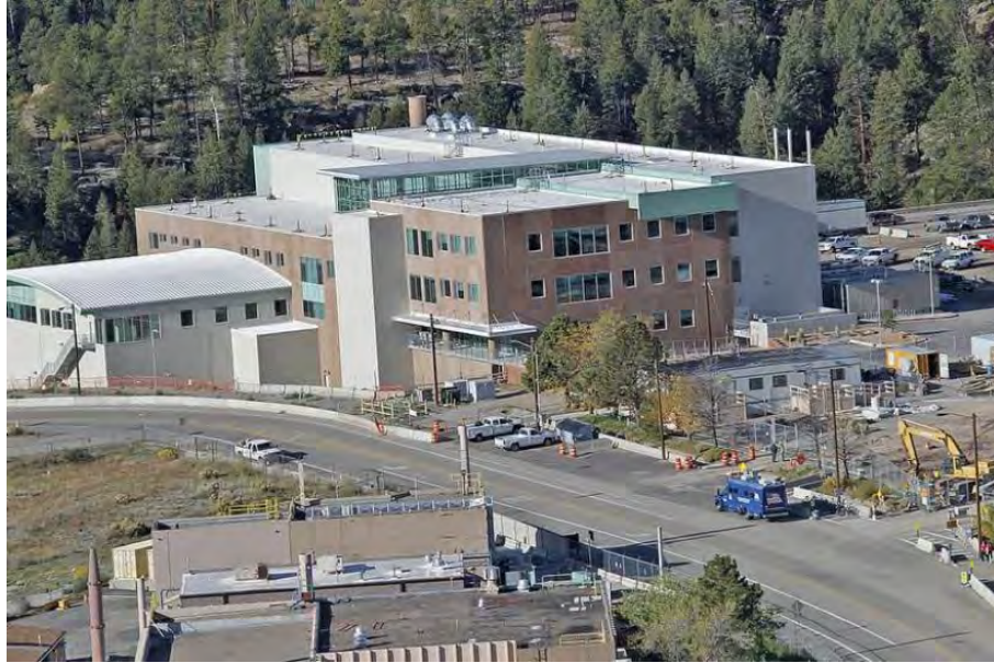
Figure 5. Radiological Laboratory Utility Office Building at Los Alamos.
