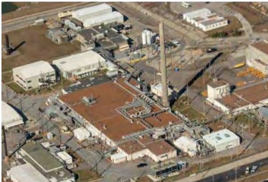
Figure 7. 296-H Stack at the Savannah River Tritium Enterprise.
