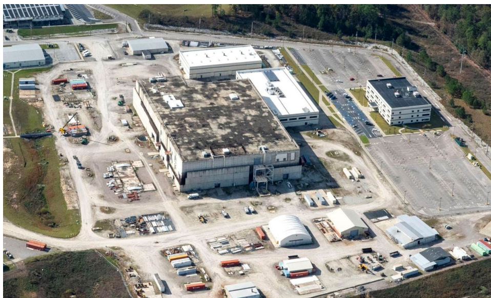
Figure 12. Savannah River Site Building 226-F
