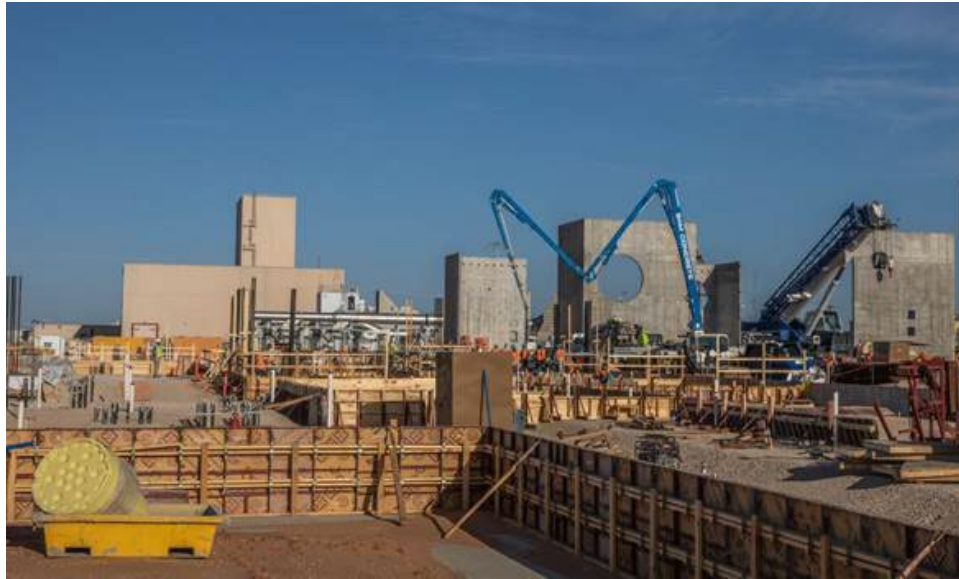
Figure 13. Safety Significant Confinement Ventilation System Construction
