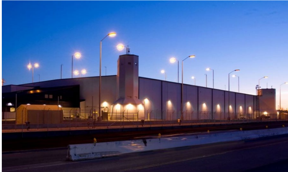
Highly Enriched Uranium Materials Facility
