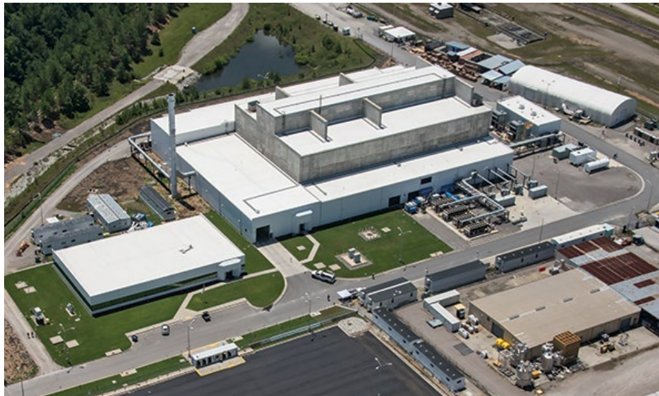
Salt Waste Processing Facility
