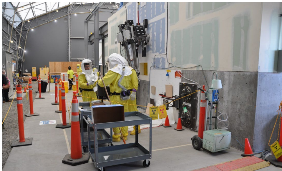
Mock-up Facility Configured for Building 324 High Contamination Area Training
