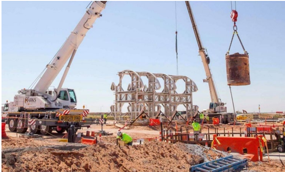
Excavation of the New Utility Shaft
