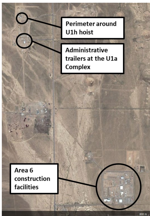
Figure 1. Aerial view of the U1a Complex and Area 6 construction facilities
