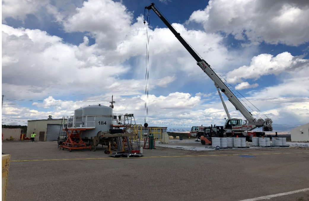
LANL Area G Mobile Loading Activities
