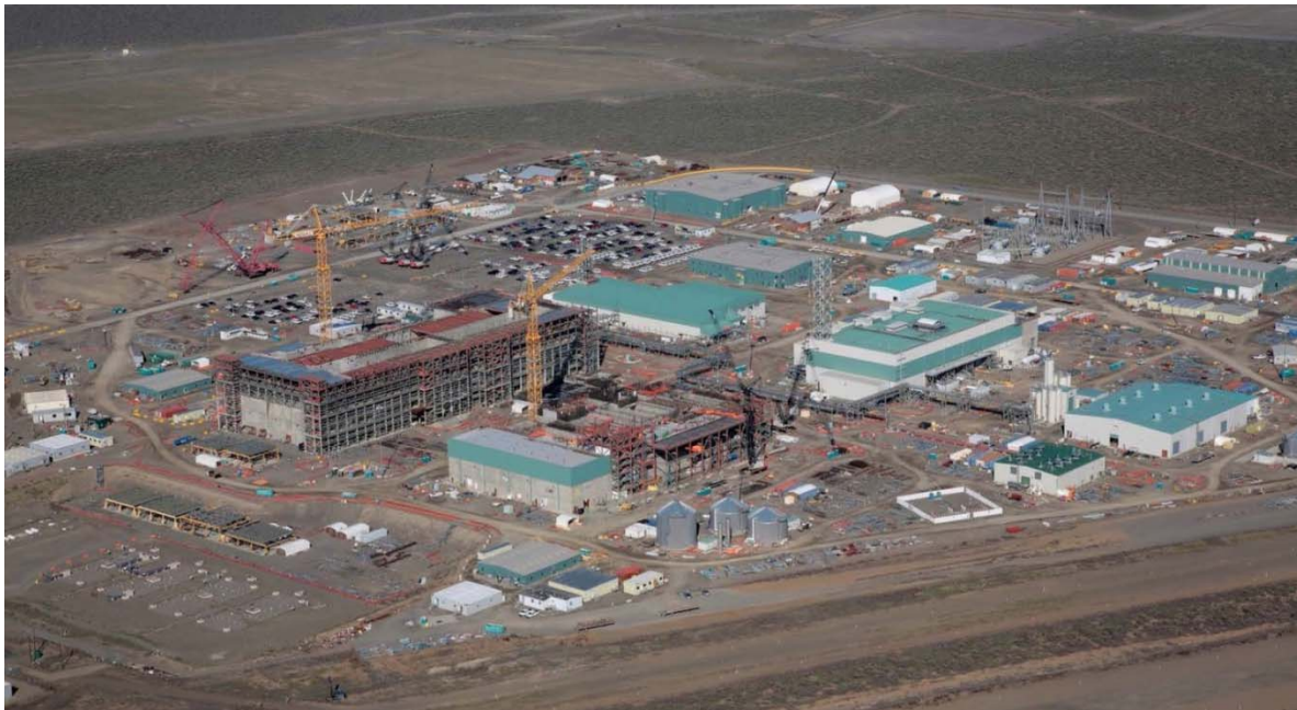
Waste Treatment and Immobilization Plant, Hanford Site
